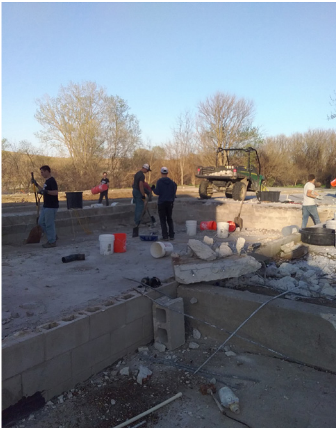
Renovation for the seminary classroom and the extension of the chapel.
