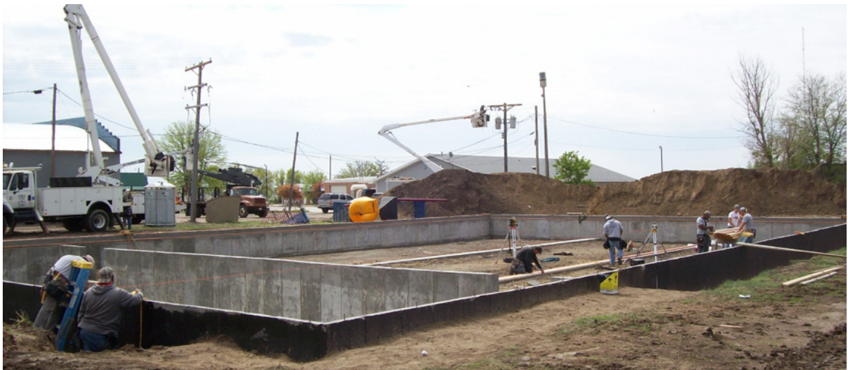
With the generous support of Immaculate Conception Church the school construction is on schedule for completion this fall
